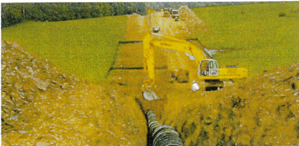
FIGURE 7: LAYING PIPE.
